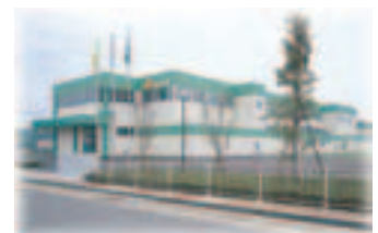
Mie Plant (TA & IT Plant)
